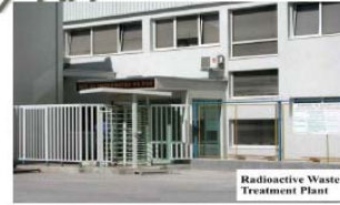
Radioactive Waste Treatment Plant
