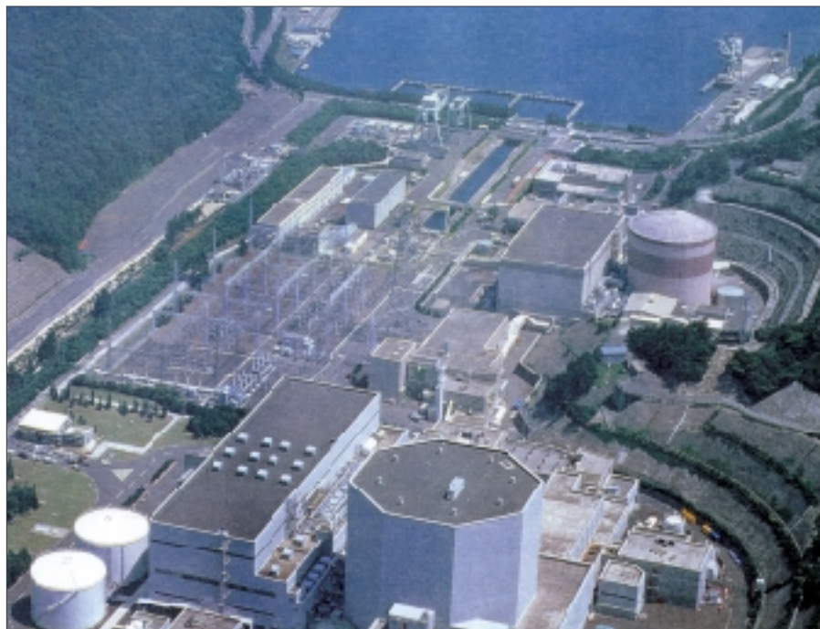
Japan Atomic Power Co., Ltd.'s Tsuruga-2 nuclear power plant, at bottom center, with its octagonal reactor building. Tsuruga-2 is an 1115-MWe pressurized water reactor. Tsuruga-1, a 341-MWe boiling water reactor, is nearby—above and to the right, with the cylindrical reactor building. (JAPC photo)
