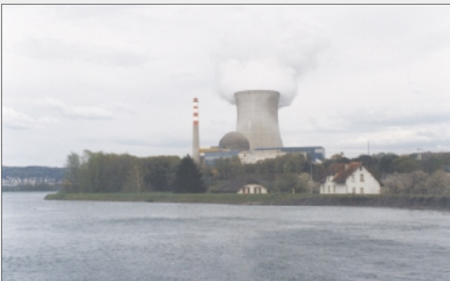
Leibstadt nuclear power station in Switzerland, across the Rhine river from two small German towns. Although the plant is located at the confluence of the Rhine and Aare rivers, it was still required to have a large cooling tower ( Nuclear News photos by Simon Rippon).
