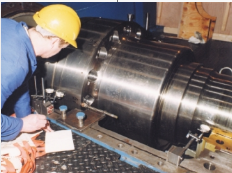
Inspecting the turbine generator at Sizewell B (Photo by Nick Davies Photography)
