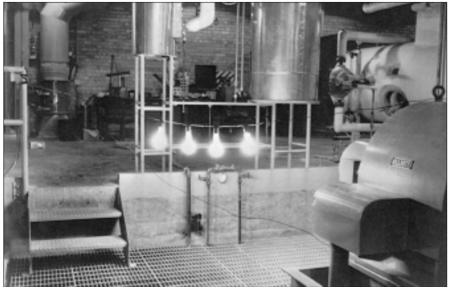
These four 200-watt light bulbs were lit up for the first time by electricity generated by nuclear power on December 20, 1951. (Source: ANL)
