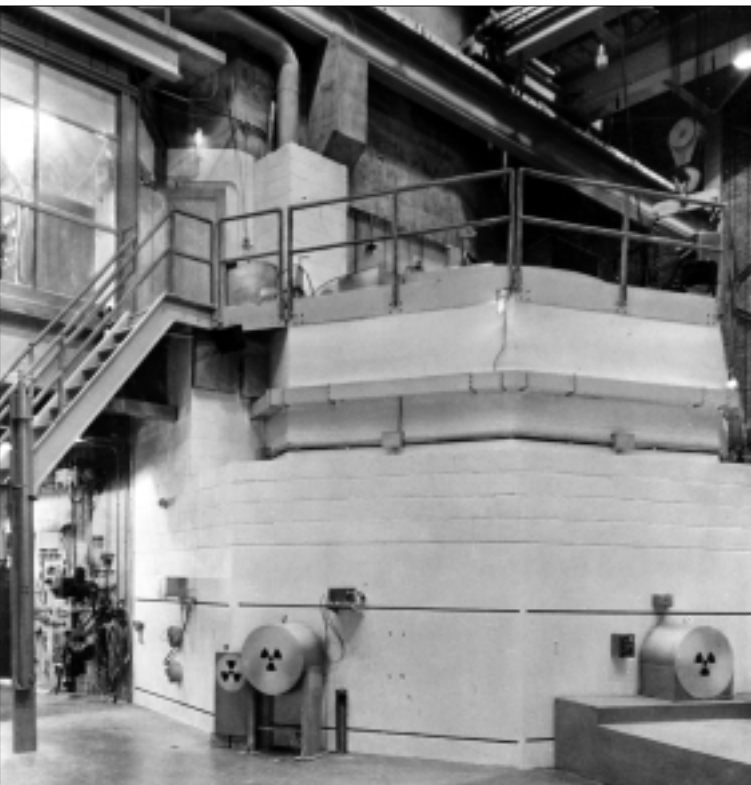
Historical photo of EBR-I reactor (Source: ANL)
