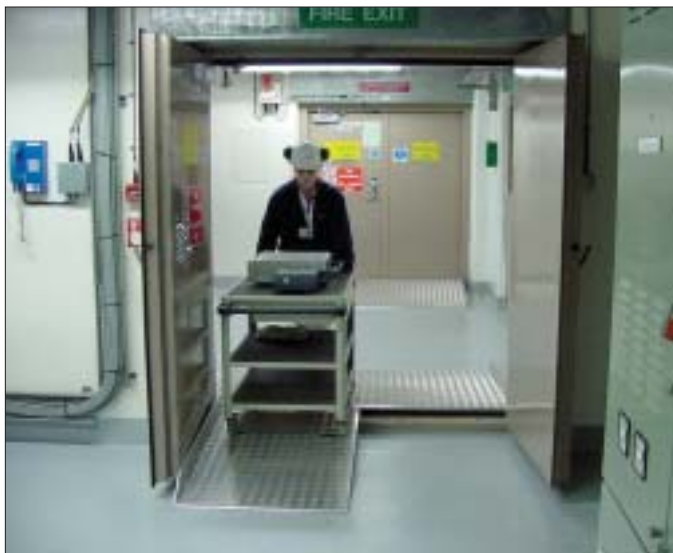
A team identified the solution of using purpose-built ramps to enable lifting trolleys for SPS/PPS (secondary protection system/primary protection system) circuit breakers to be moved over a high-integrity fire door with a large step built into it. (BE)
