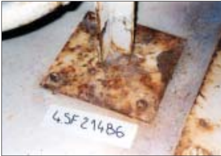
Corrosion and aging phenomena—as shown in the photos above—if unrecognized, can put the plant at risk. (EdF)
