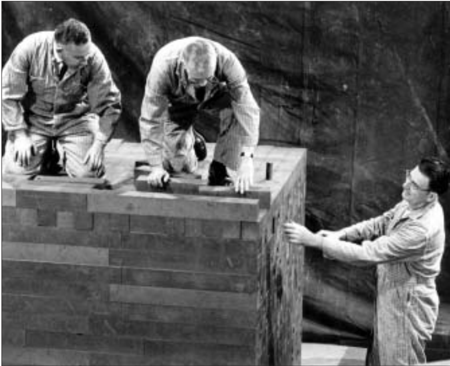
Workers assembling CP-1 (Photo: Argonne National Laboratory)
