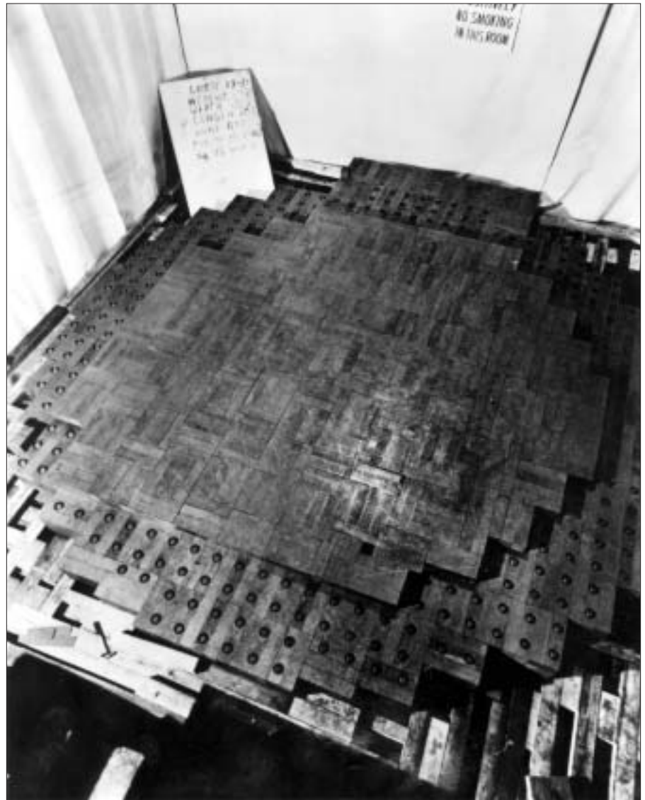
Photo of CP-1 during construction, before layer 19 was complete. Pure graphite layers like layer 19 alternated with layers of uranium dioxide "pseudospheres" embedded in graphite, such as can be seen on the exposed edges of layer 18. Parts of the wooden scaffolding and surrounding balloon cloth also are visible. (Photo: ANL)
