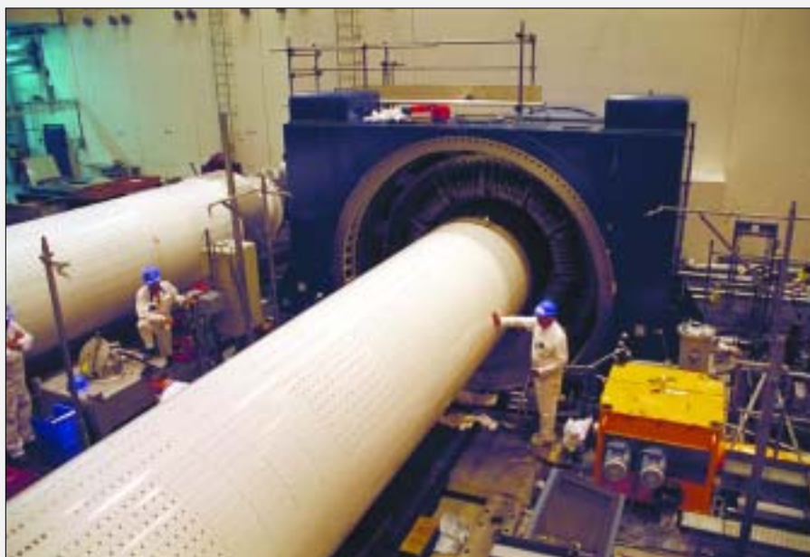
A generator rotor being exchanged with a spare in order to equalize operating hours on each, at Forsmark-3 (Photo: Odd Hedberg/Forsmark)
