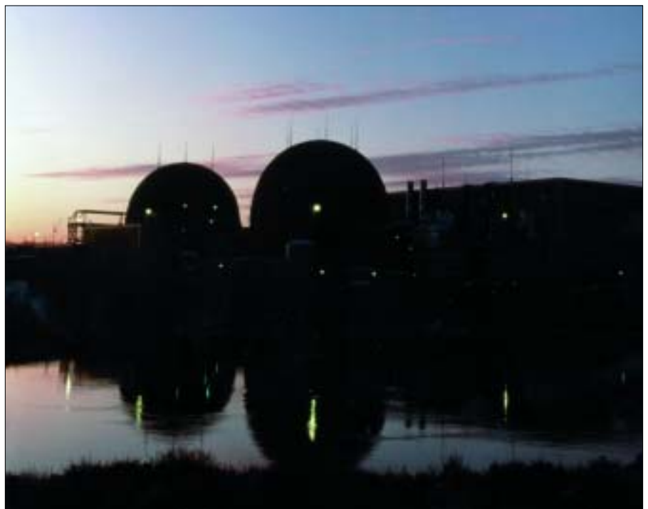
North Anna: Possible site for a new Dominion reactor
