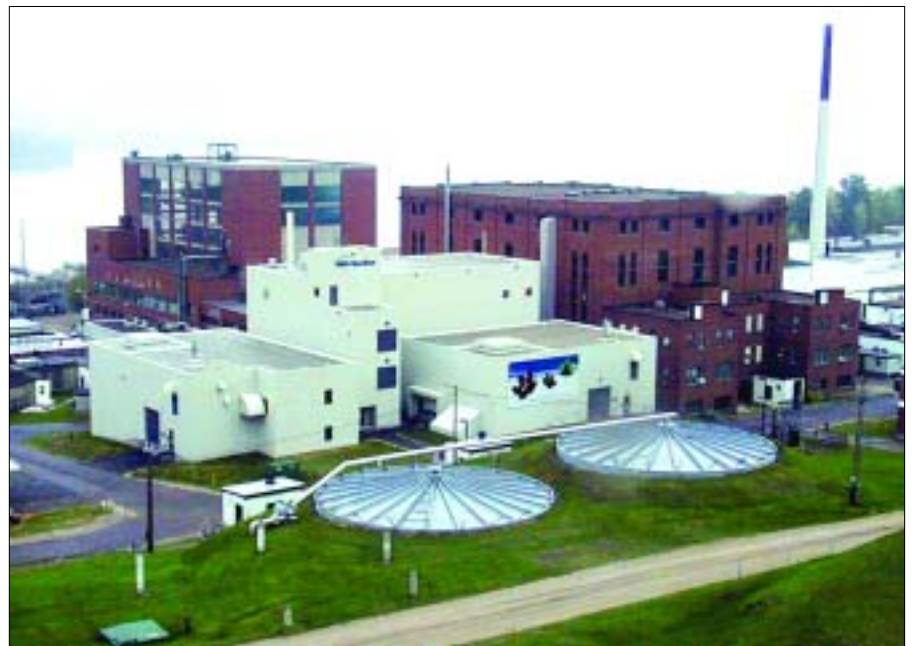
MAPLE reactors: Unit 2 (white building on left) and Unit 1 (white building on right)
