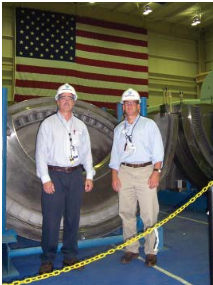
Steve Sarver (left) and Skip Jordan: On the turbine deck at the Millstone-2 nuclear power plant. Behind them is a new turbine that will replace an existing component during an outage in October.
