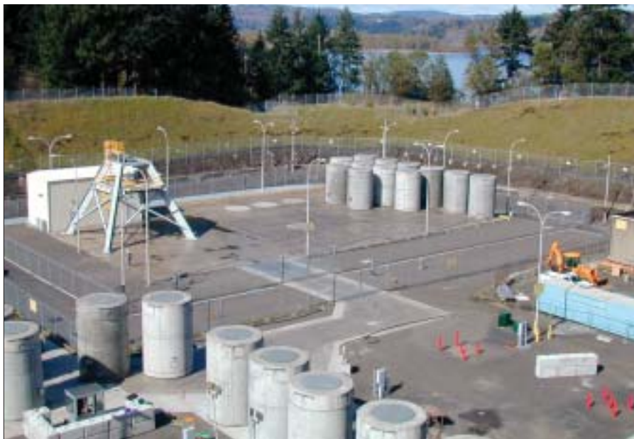
ISFSI pad with loaded casks at the Trojan plant (PGE)
