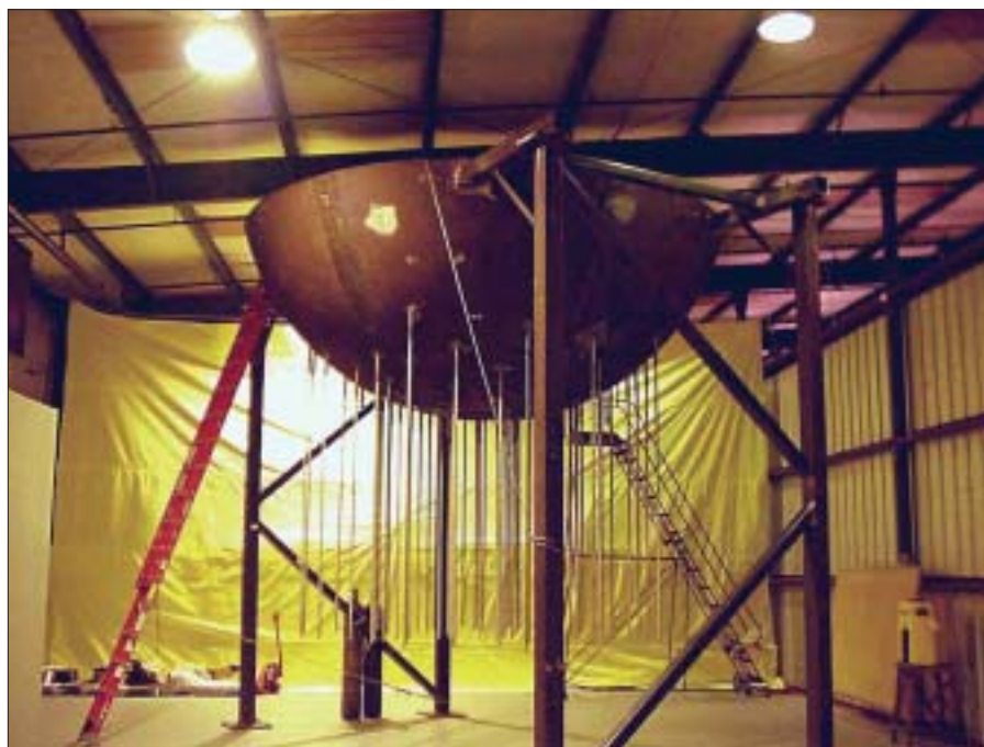
A mock-up of the lower half of STP-1's reactor vessel was used on-site by workers to practice various tasks before the real repair job was done. The long pipes descending from the reactor are instrumentation tubes. (Source: STP Nuclear Operating Co.)
