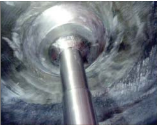
A close-up of a repaired nozzle, which was secured to the outside of the reactor by welding it to a thick, nickel-chromium pad. (Source: STP Nuclear Operating Co.)
