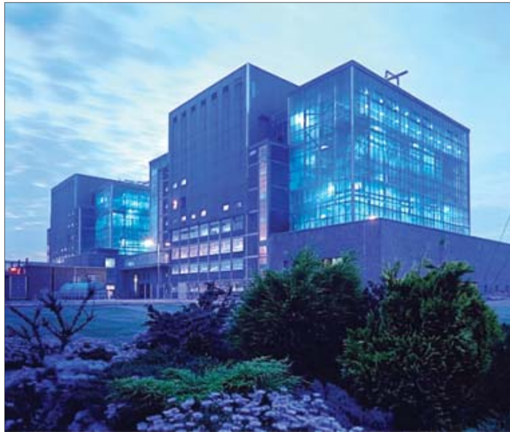
The Bradwell nuclear power plant
