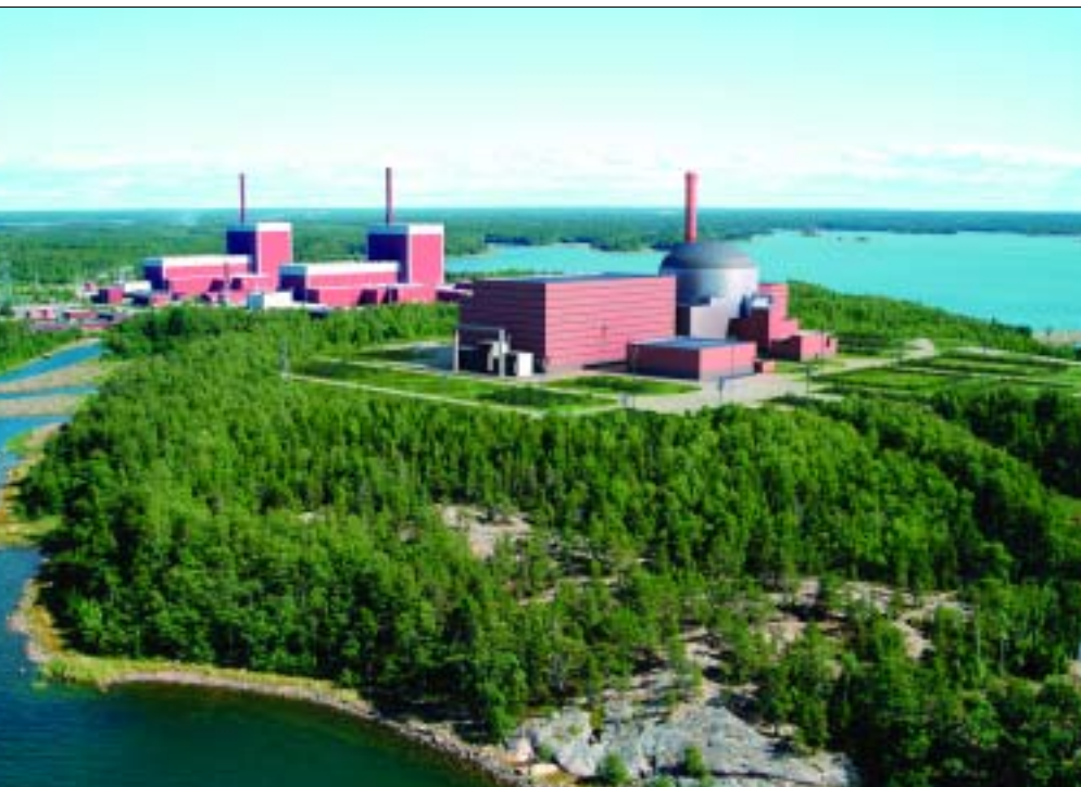
Fig. 5. Artist's conception of the first EPR that will be built, Olkiluoto-3 (foreground), on the site with Olkiluoto's two currently operating units.
