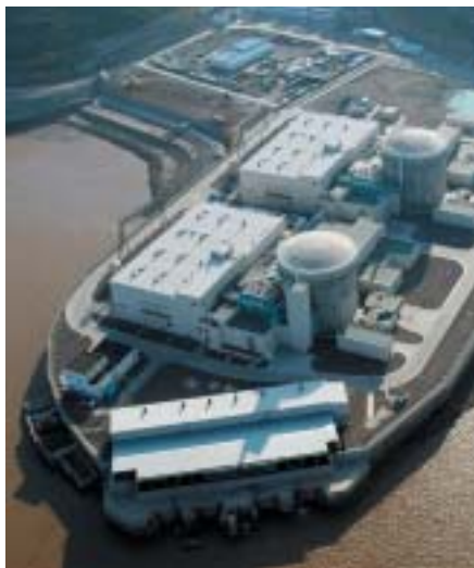
Two CANDU 6 units at Qinshan, China
