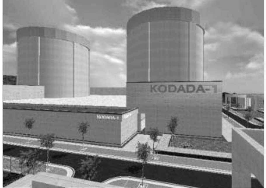
The KODADA-1 nuclear power plant can be accessed from a computer located anywhere in the world, provided there is an Internet hookup.
