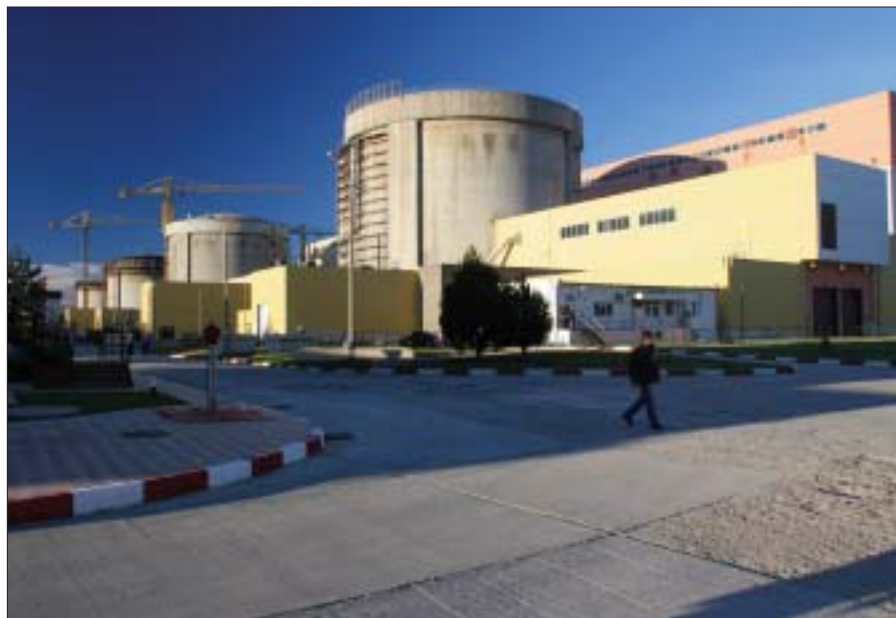
Cernavoda: Construction is now well advanced on Unit 2.
