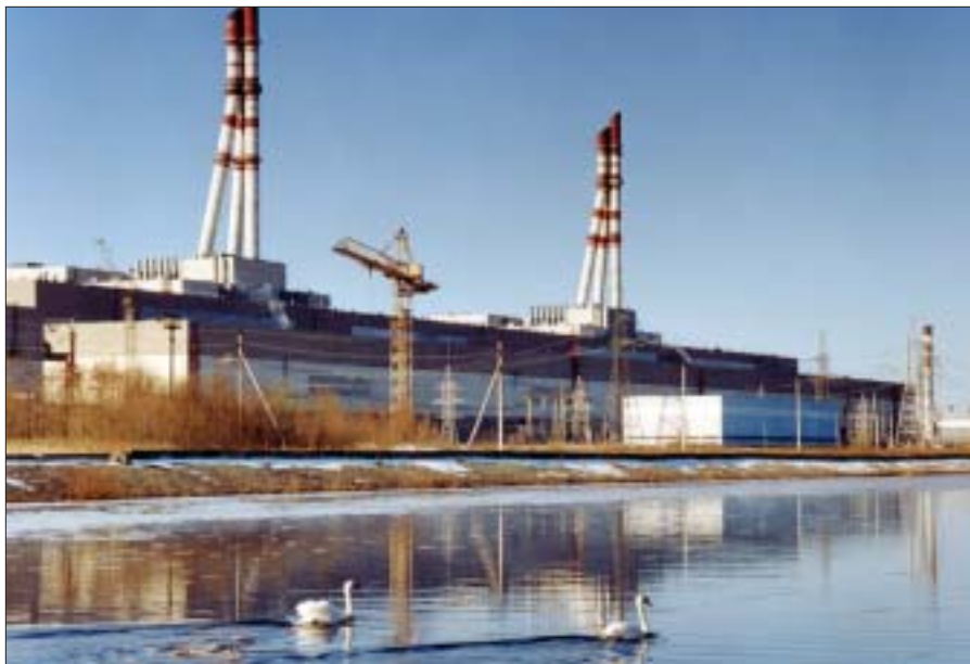
Ignalina: The planned closure of Unit 2 in 2009 is now being rethought by some officials.
