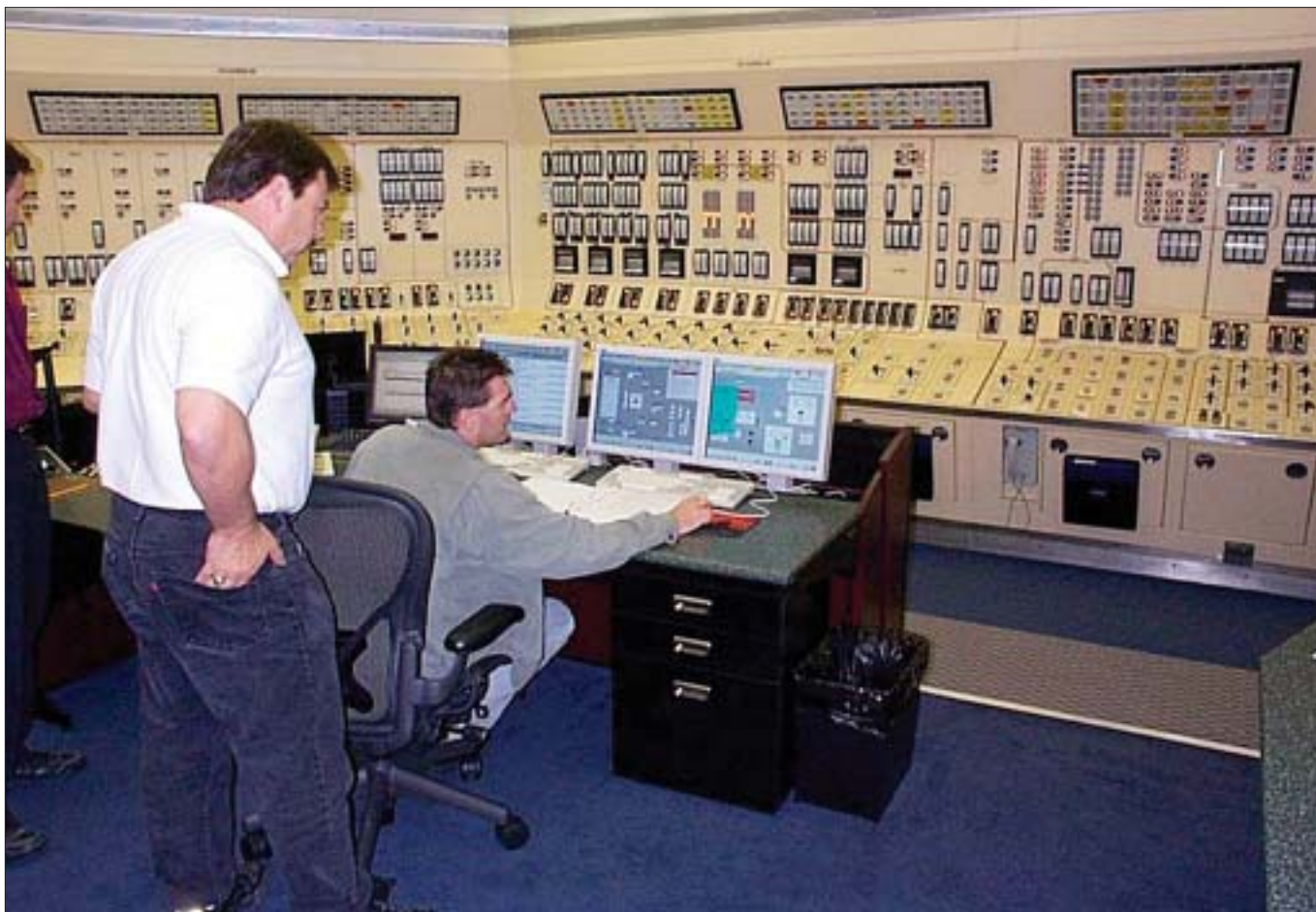
Comanche Peak operators receive training on the new digital Turbine Generator Control System in the plant's simulator. The displays shown are the same as those installed in the actual Comanche Peak control room. (Photo: TXU Power)
