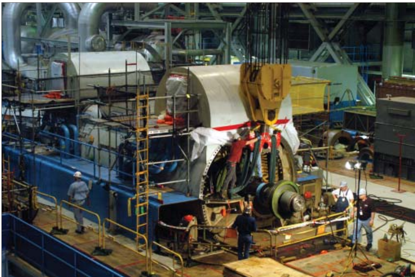
Maintenance work on the main generator during the spring 2004 outage
