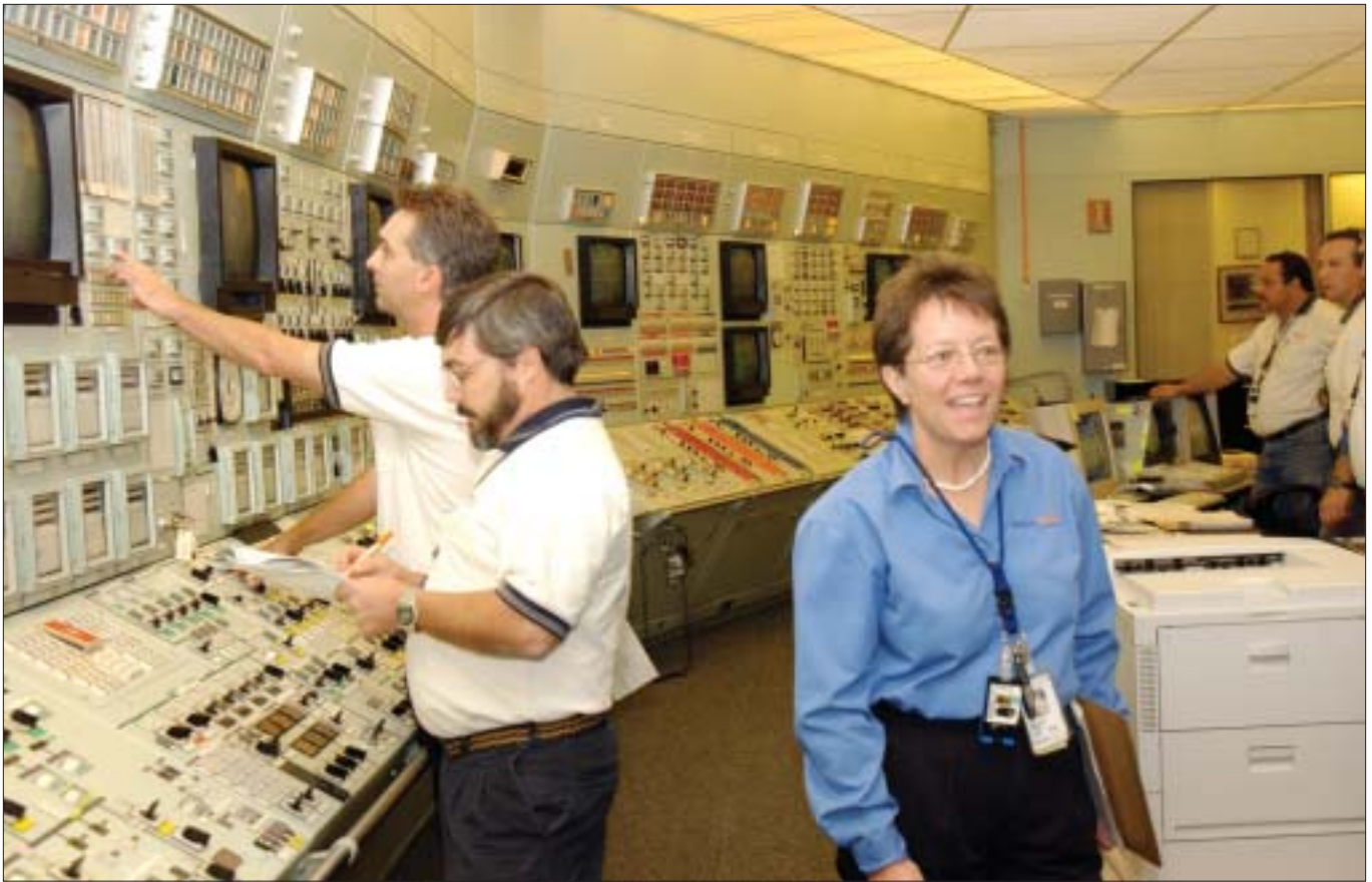
Shift Manager Carol Lenestour (right) announces the synchronization of Bruce-4 to the Ontario electricity grid on October 7, 2003, ending an outage that lasted more than five years. (Photo: Bruce Power)
