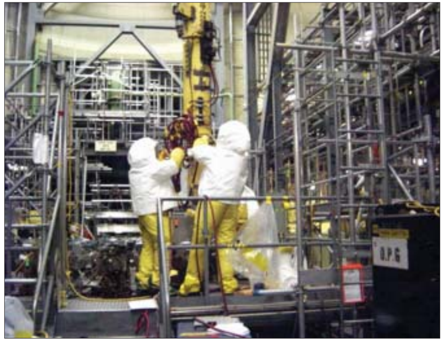
A 10-ton flask is positioned at Pickering-1 as part of the shutdown system enhancement. (Photo: Ontario Power Generation)
