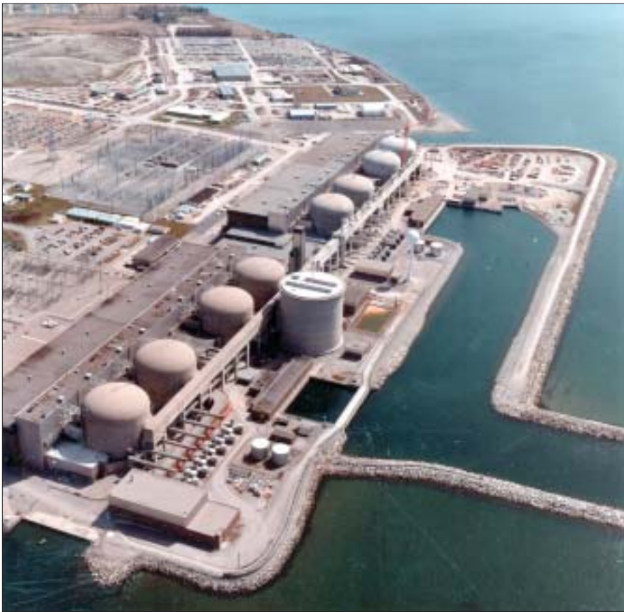
Pickering-1, fourth from left, went critical in August, and will soon join Unit 4 (left) and Pickering B (the four units at right) in power production. (Photo: Ontario Power Generation)
