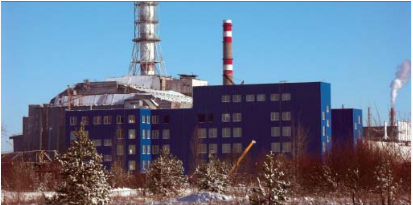
In the foreground, a new clothes-changing facility for contractors involved in the Shelter transformation activities. In the background, Chernobyl-4 enclosed in its sarcophagus. (Photo: Insight )
