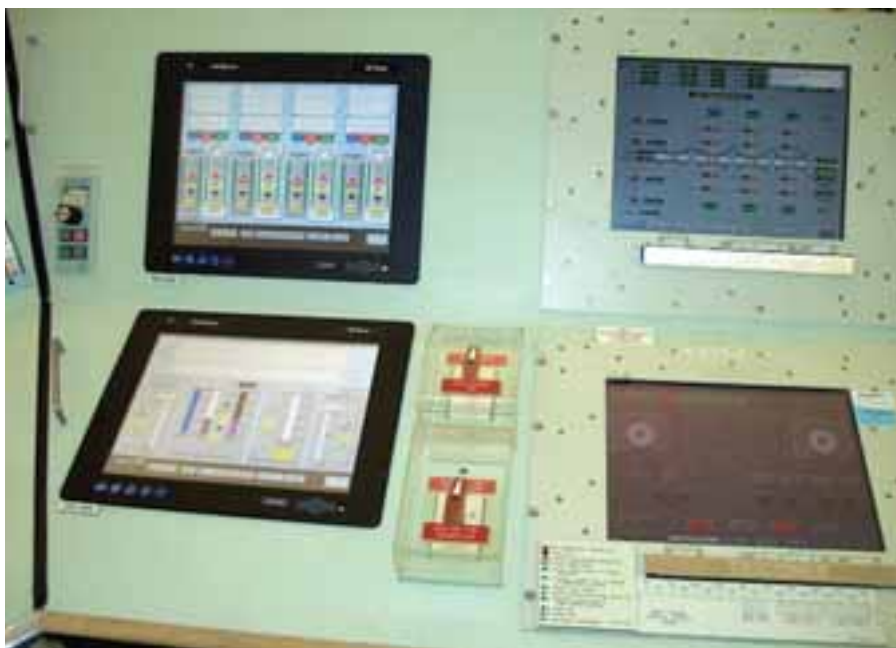
Diablo Canyon's two control rooms were retrofitted with digital soft control human-machine interfaces such as these for feedwater and main turbine control systems. (Photos: Scott Patterson)
