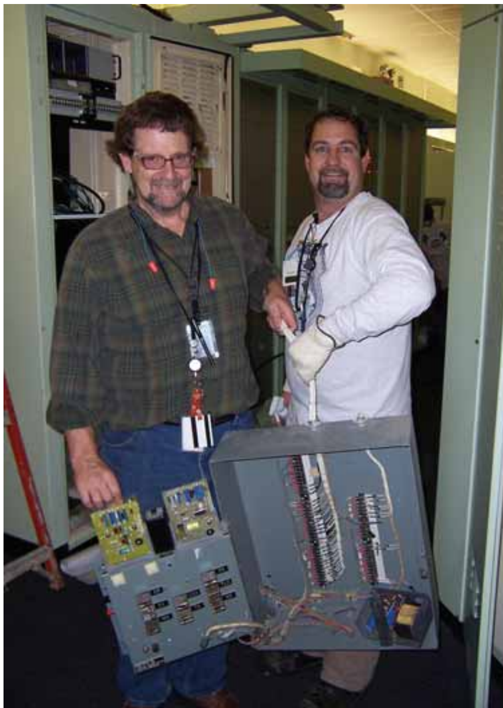
I&C technicians Jeff Carter and Mark Machala remove old analog equipment from the moisture separator reheat system before replacing them with new digital components.
