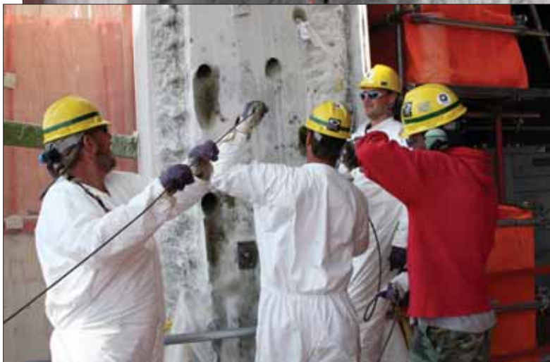
Above & Inset: In order to cut the opening in the containment building, workers use jackhammers to remove the final few inches of concrete surrounding the rebar that is part of the containment's liner.
