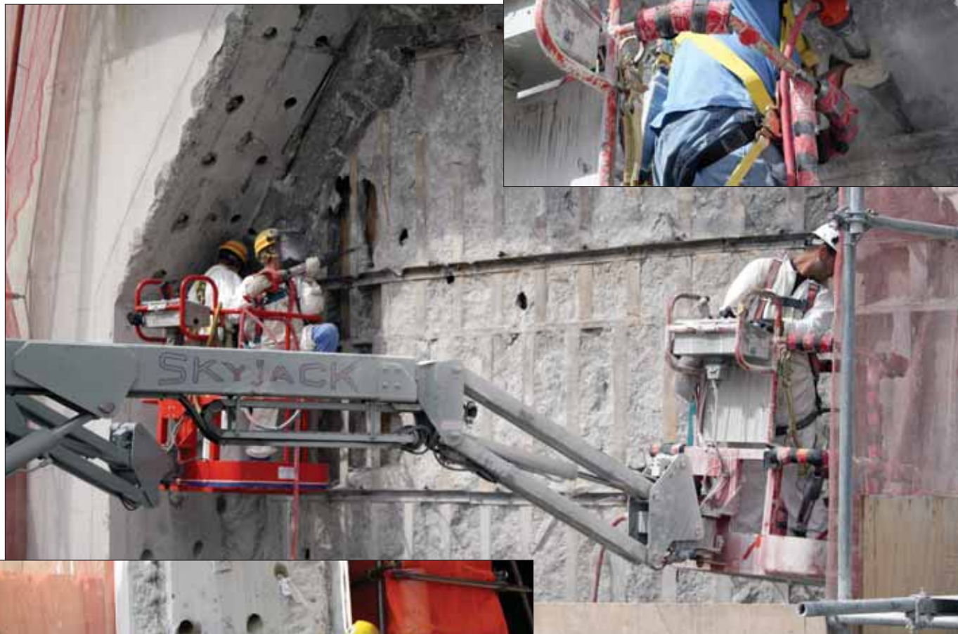
Above & Inset: In order to cut the opening in the containment building, workers use jackhammers to remove the final few inches of concrete surrounding the rebar that is part of the containment's liner.
