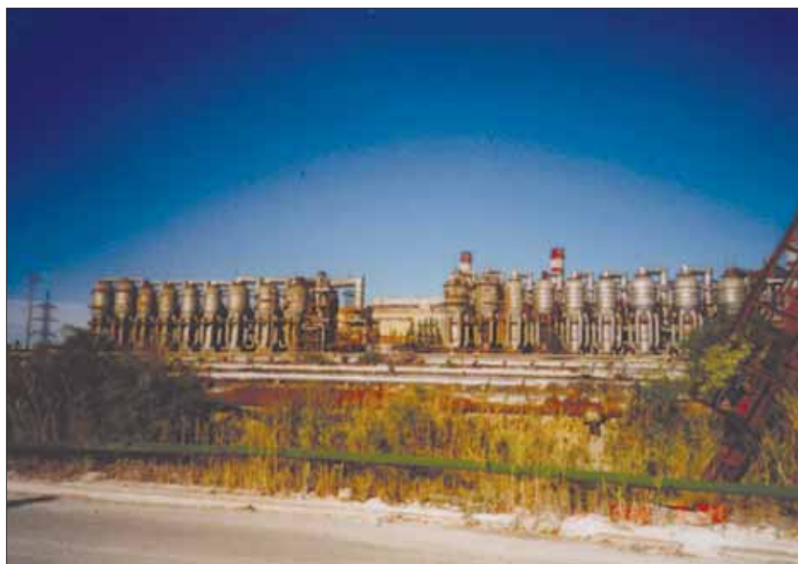
The desalination plant evaporators at Aktau, Kazakhstan. The BN-350 fast reactor at Aktau supplied potable water to local communities until it was shut down in 1999. (Photo: IAEA)
