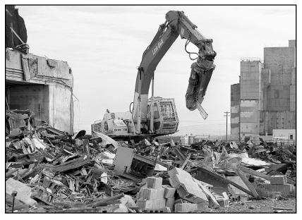
Demolition began in February at Hanford's fourth plutonium production reactor to undergo the cocooning process and should be completed in fiscal year 2003. In the background is DR Reactor, where cocooning is 85 percent complete. The final step in the DR Reactor cocooning process is to install a new roof over the entire structure, which should be completed in fiscal year 2002. Hanford is home to nine surplus plutonium production reactors.
