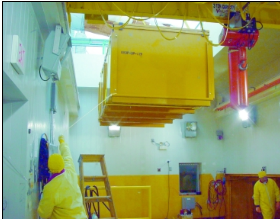
A mobile crane was used to lift out the waste containers from the enclosure for placement in storage and eventual disposal.
