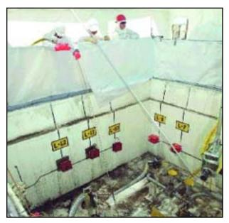
Compared to baseline pit operations methods shown here, remote systems will reduce worker exposure and enable more thorough removal of discarded materials in Hanford pump pits. (Photo courtesy ORP.)
