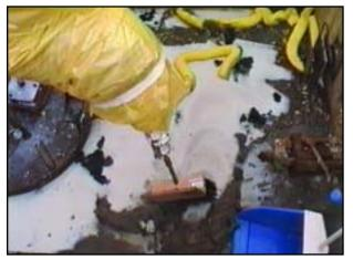
A brush tool was attached to the Pit Viper manipulator arm to scrape and scoop debris from the floor of the Tank C-104 pit. This was the final of five required tasks (size reduction and foam removal, wall spraying, wall grinding, scraping/scooping, and debris removal) to demonstrate the system's capabilities in a highly radioactive environment.
